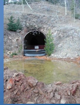
Big Five adit -Ward, CO
