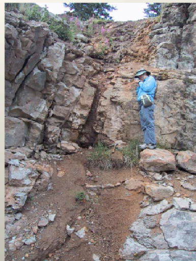
Fault Trace – In Vicinity of Koehler Tunnel Drainage
