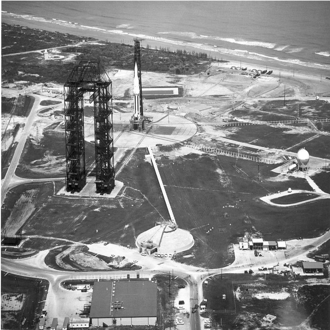
Figure 4-31. Aerial view of LC34. Engineering Support Building, bottom of photo.
