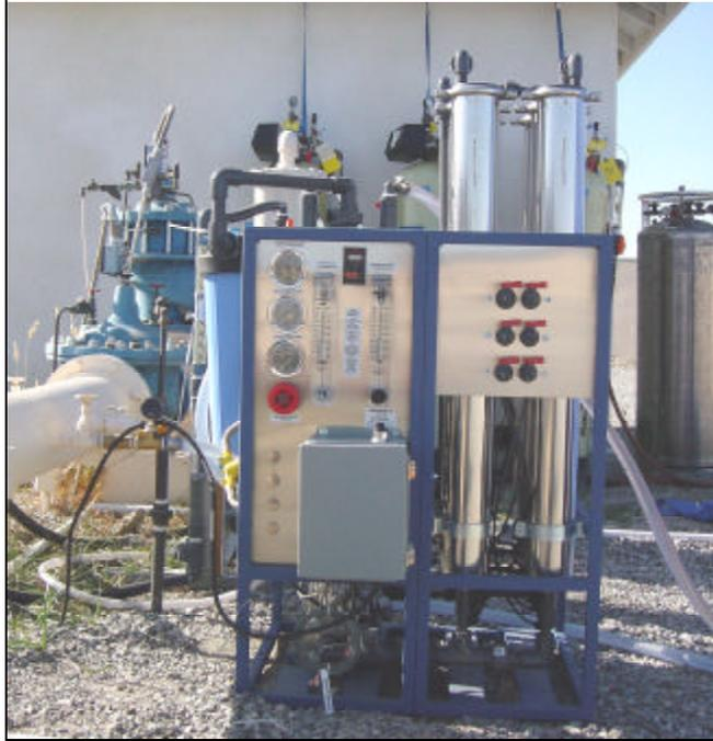
**Photograph 2: Watts Premier M-15,000 RO Treatment System at CVWD Well 7802**
