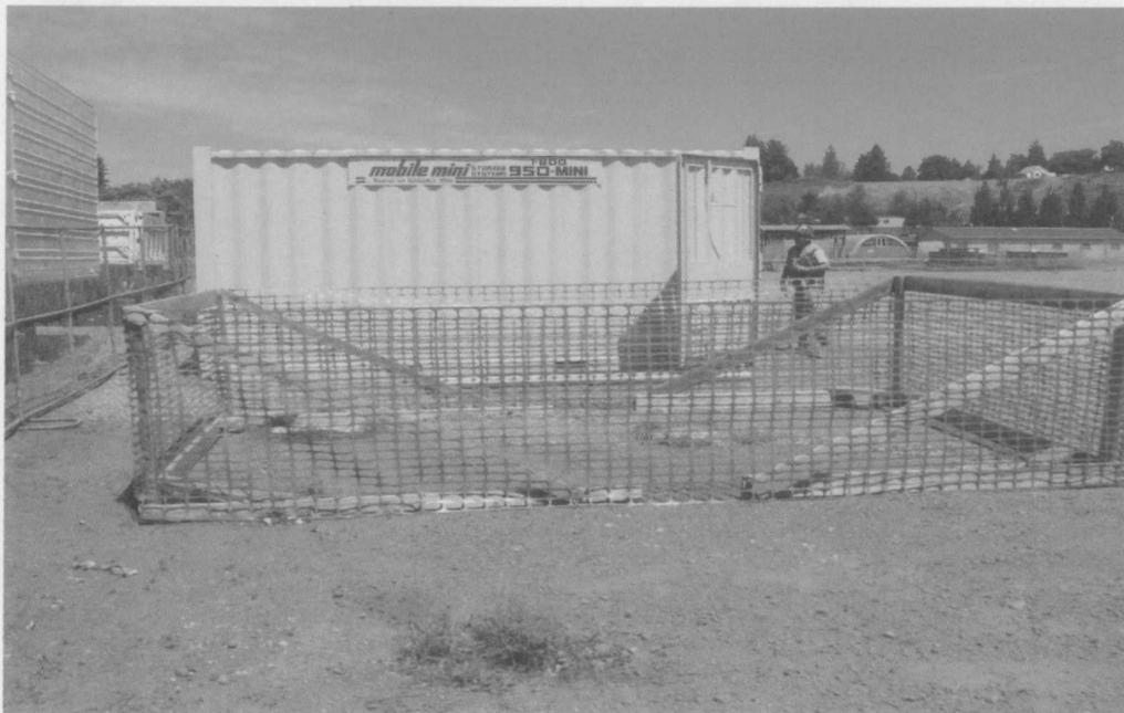
Figure 3.0, looking north near the former FHC site shows how the wells were being protected during the construction/development work. Wells inside the corral are inj-1, 2, MW-7, and MW-1.
