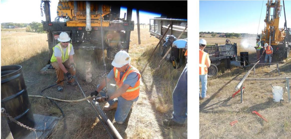
**Figure 3-24. Application of hot water to the cooling coils to release the sample liner**
