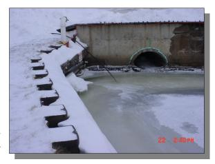
Ice soundings were conducted twice in the month before field work started, on February 18 and 24, 2004 (Appendix A, ice soundings). The soundings revealed an ice thickness greater than 12 inches across the Slip on February 18, and a thickness of at least 18 inches by February 24. Though the ice was not consistently thick enough to support a truck-mounted probe, it was sufficient for the smaller track-mounted probe, which was the approach selected for this project.
