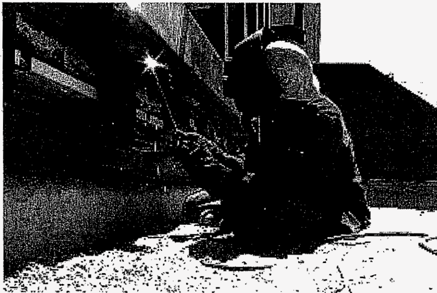
Figure 2.3-17 Block Stop Installation
