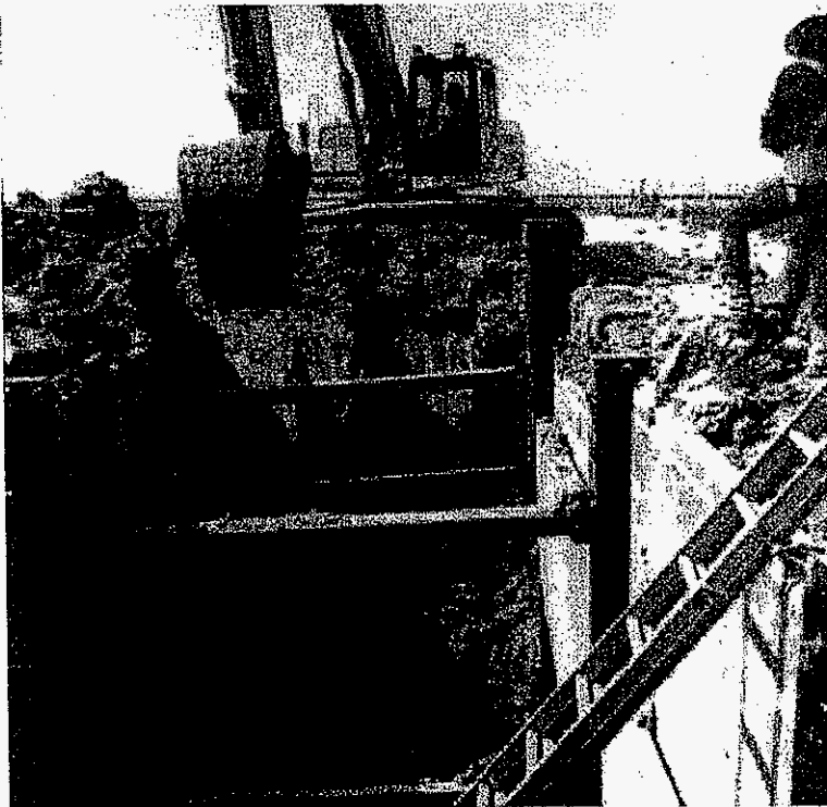
Figure 2.1-3 Slide-Rail Shoring System
