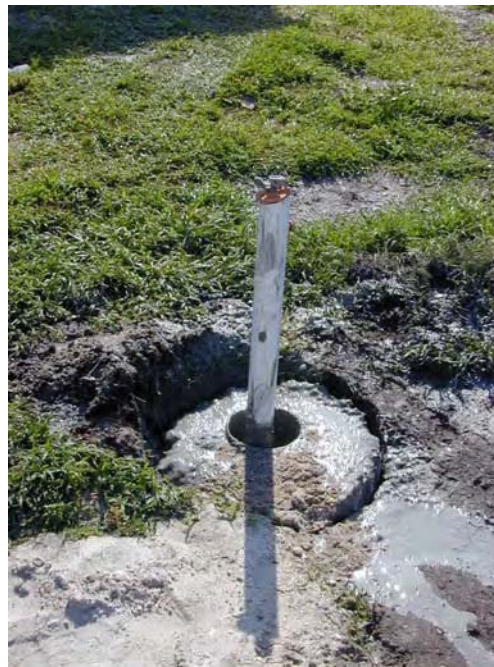
Figure 4-11. Pictures Showing (a) Installation of the Surface Casing and (b) the Completed Dual-Casing Well
