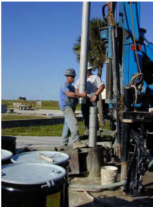
Figure 4-11. Pictures Showing (a) Installation of the Surface Casing and (b) the Completed Dual-Casing Well
