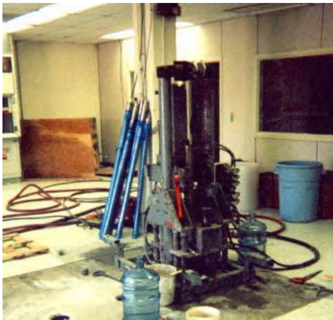
Figure 4-5. Indoor Vibra-Push Rig (LD Geoprobe® Series) Used in the Engineering Support Building
