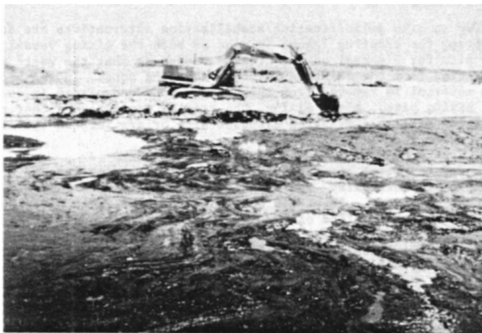
Figure 6-3. In-situ mixing with a backhoe at a large site. (Courtesy Albert H. Halff Associates)
