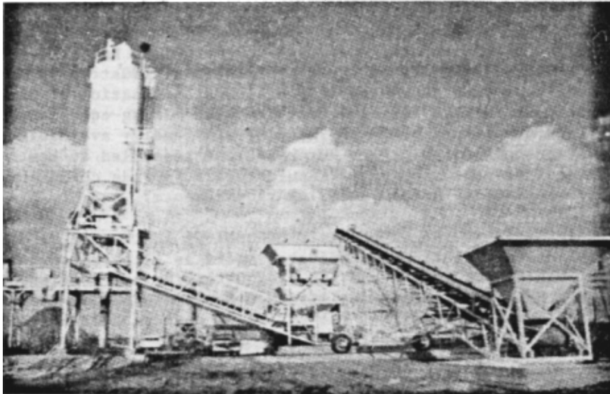
Figure B-11. Typical base stabilization plant.
