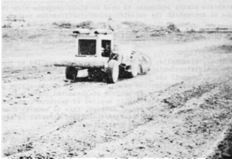
Figure B-10. Typical high-speed rotary mixer (Courtesy Albert H. Half Associates).
