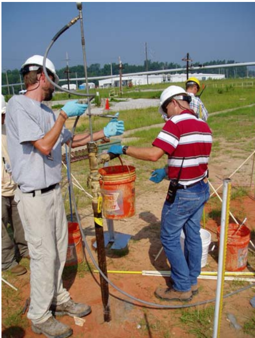
Figure 5 – Notching Well Prior to Hydraulic Fracturing
