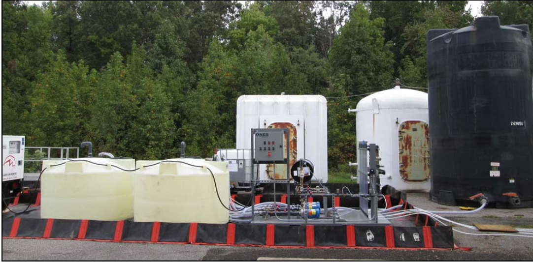
Figure 6.3: Injection Skid Assembly with all Components
