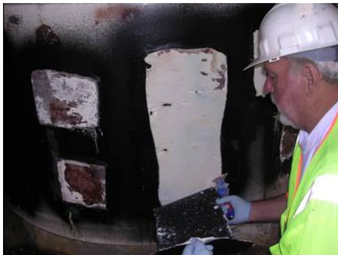
Figure 57. Sampling of large tank NM-VP, three weeks after application.
