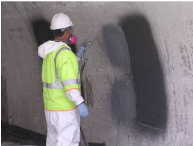
Figure 6. Silicon sealant application with spray gun.
