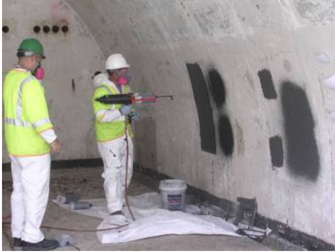
Figure 5. Vinyl polymer sealant application using spray gun.
