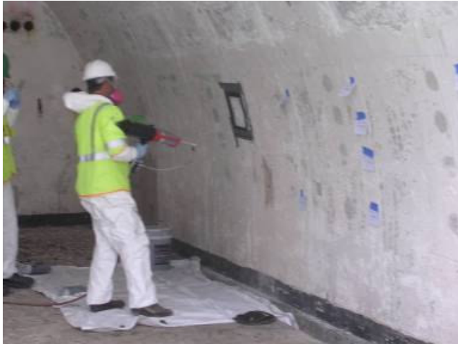
Figure 3. Spraying BTS with cartridge-type spray gun.
