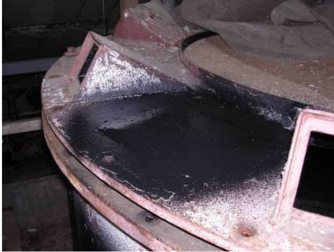
Figure 46. Large tank lid, treated with MgPd-VP, immediately after application.
