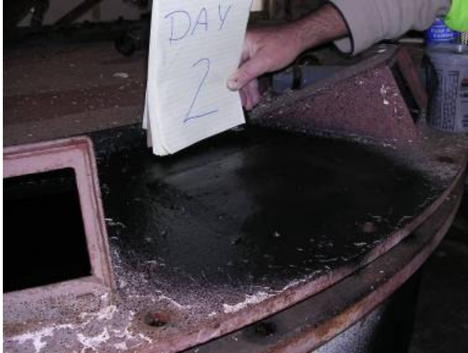
Figure 48. Large tank lid treated with MgPd-VP, two days after application.
