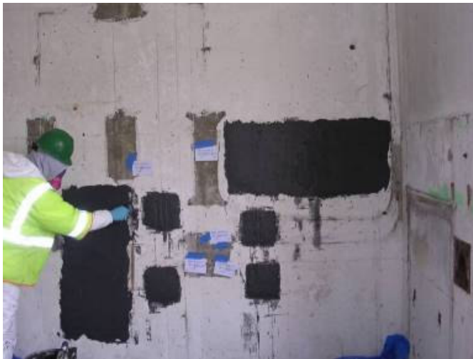
Figure 27. Application of MgPd BTS prior to sealing with vinyl polymer or silicon sealant, 6810-36.
