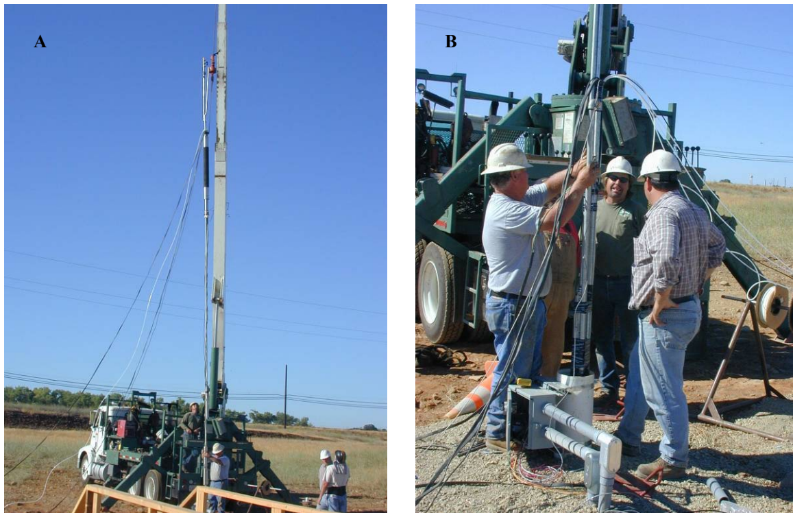
Figure 3. Photograph of equipment installation into the downflow HFTW at Aerojet. The packer is visible in photo A, and the wiring, tubing, and equipment present in the HFTW is seen in photo B.
