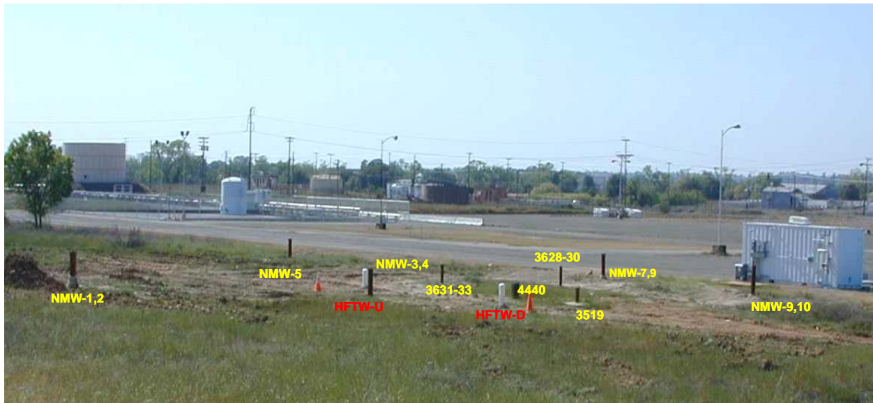
Figure 5. Photograph of the Aerojet HFTW system showing location of HFTWs and all monitoring wells.
