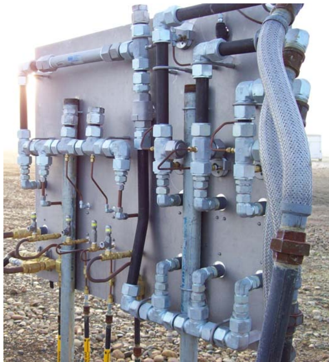
Figure 7 – Gas Supply Control Panel
