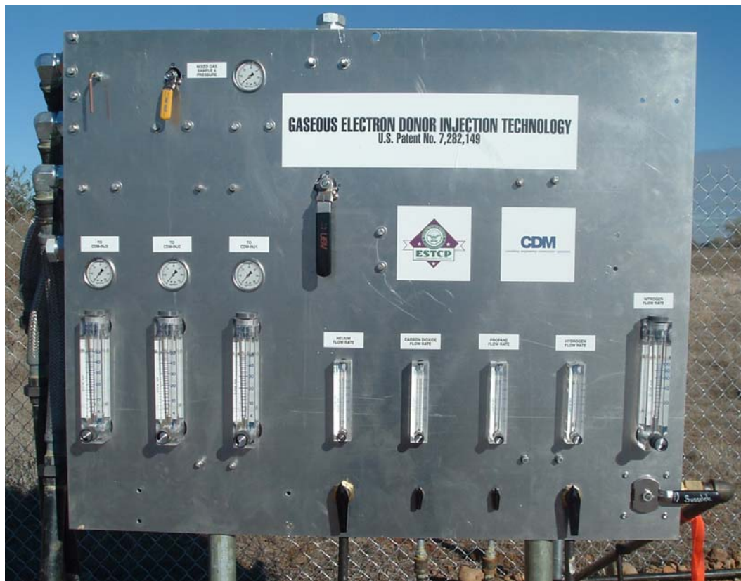
Figure 31 – Gas Supply Control Panel
