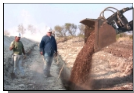
PRB Installation at NWIRP McGregor
