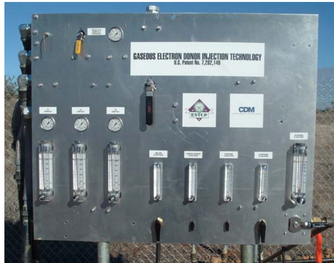
Figure 8. Gas supply control panel.
