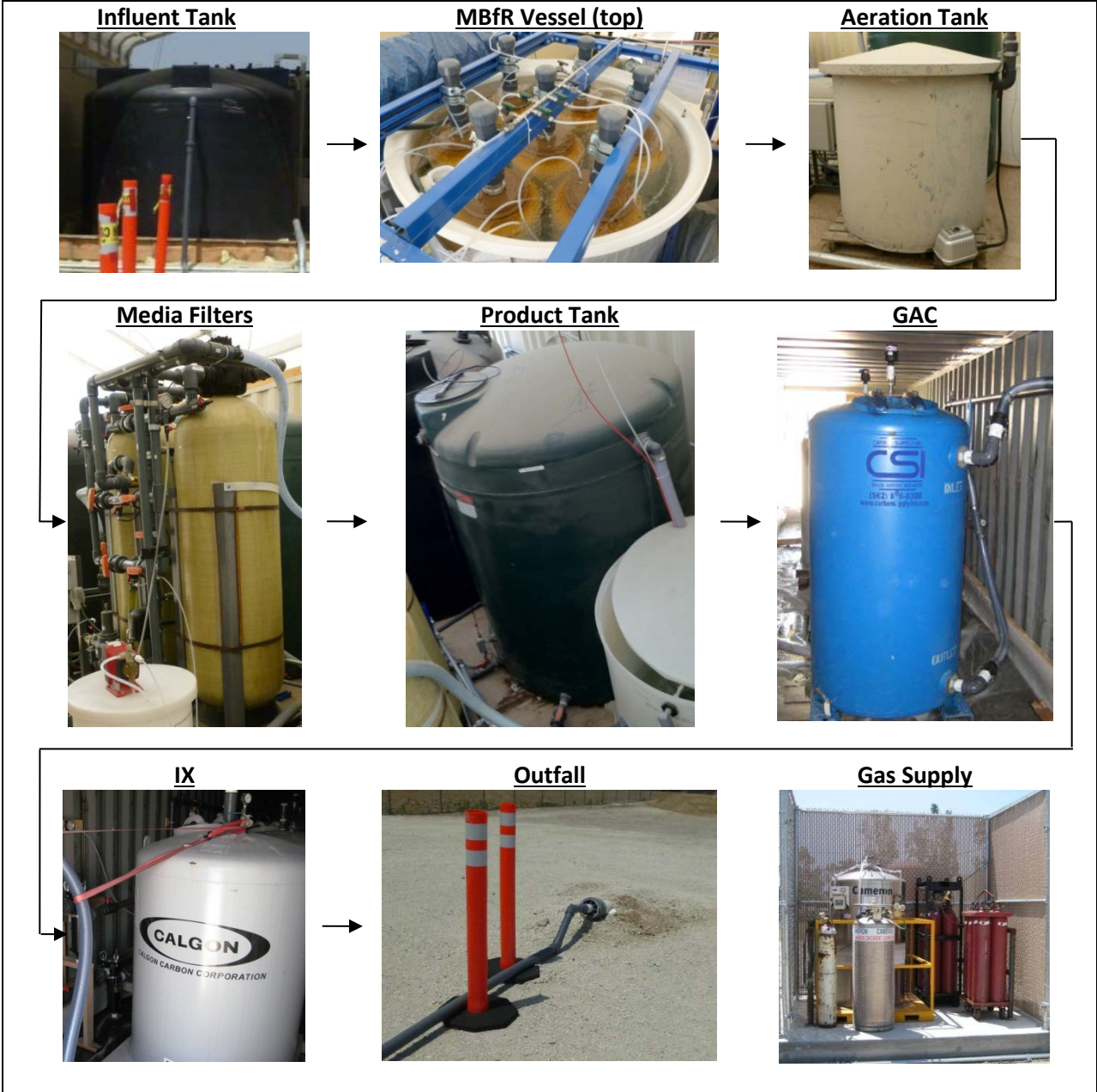
Figure 5.4 MBfR Treatment System Process Flow
