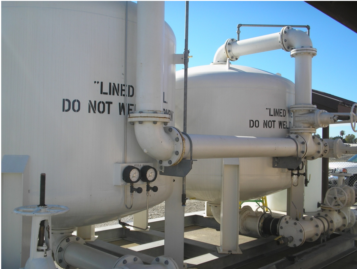
Figure 12. Face piping and well connection – WVWD.
