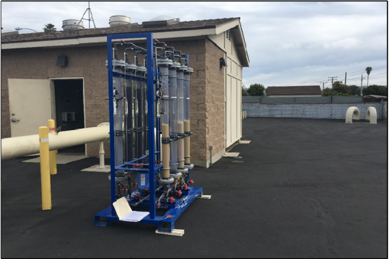
Apr 17, 2020, Treatment skid following delivery to the site by AqueoUS Vets.
