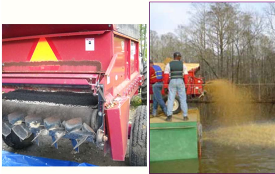
Figure 10. Barge-mounted TurfTiger spreader. The picture on left shows on-land delivery trial for SediMite ® ; picture on right shows a thin-layer sand cap spreading operation that was essentially the same deployment approach used for SediMite ® delivery to LCC.
