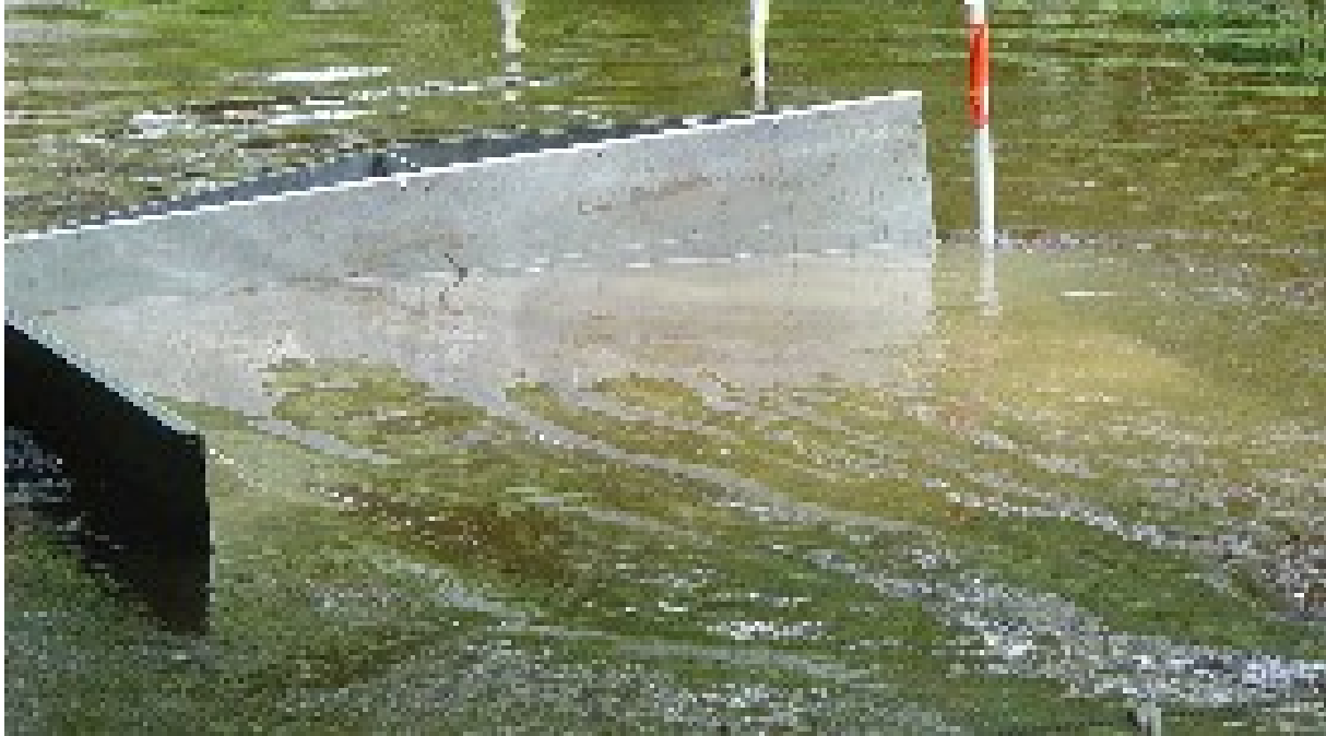
Picture 9. Cap Frame was Removed in Sections after Cap Construction was Completed.
