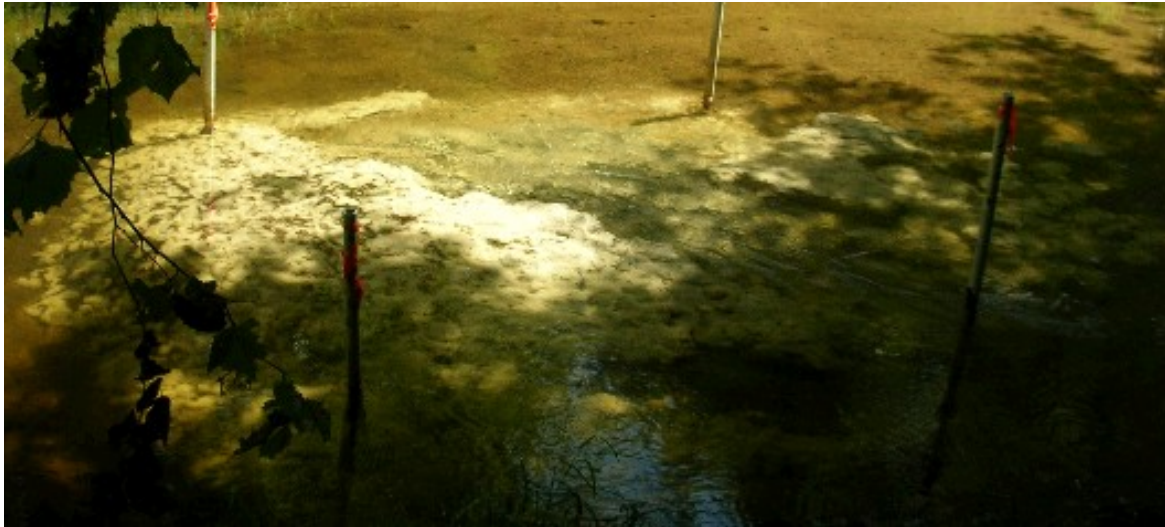
Picture 19. Plot 8 – Three-layer Cap Composed of Biopolymer/Sand Slurry, a Two Inch Middle Layer of 50% Apatite and 50% Sand, and a Two Inch Bottom Layer of 25% Organoclay and 75% Sand.
