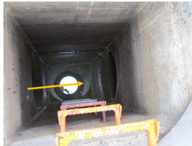
Orange arrow indicates direction of flow. Pipe submerged approximately halfway in standing water. Standing water in pipe indicates potential tidal influence. Pipes appeared to be concrete and did not appear to be slip lined.
