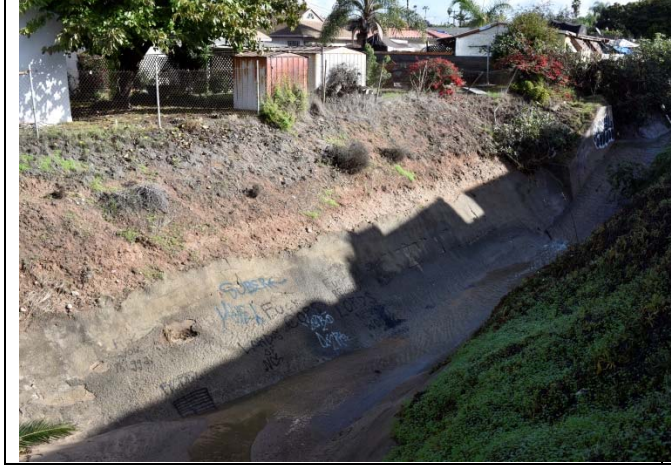
Concrete-lined channel, but bare dirt and poor vegetation above concrete that are erosion sources. Some scoured silt/clay on bottom of channel evident. Some new erosion on bank side.
