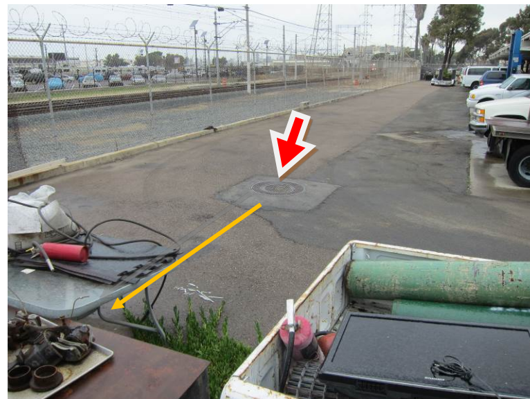
Recommended sampling location at the manhole located northwest of Outfall Location #3. Orange arrow indicates direction of flow. MS4 map review and site reconnaissance indicates this is the last storm drain access point prior to entering Paleta Creek.
