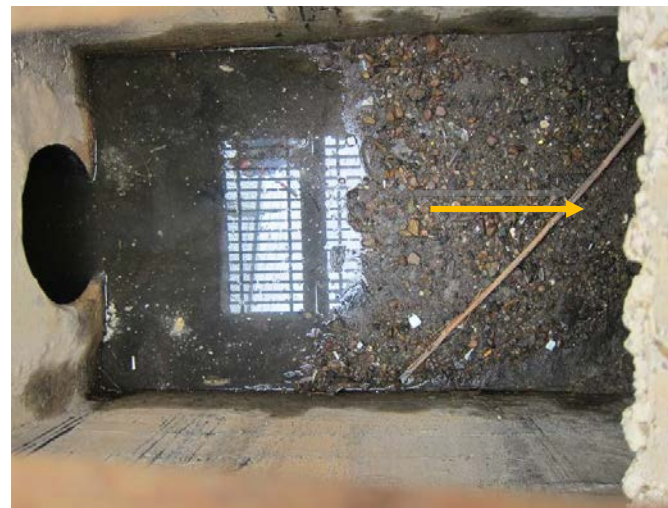
Tidally influenced catch basin. Orange arrow indicates direction of stormwater flow. Upstream pipe is slip lined PVC/HDPE. Downstream pipe is corrugated metal (CMP). Rocks (approximately 1" diameter), sediment and sand in catch basin.
