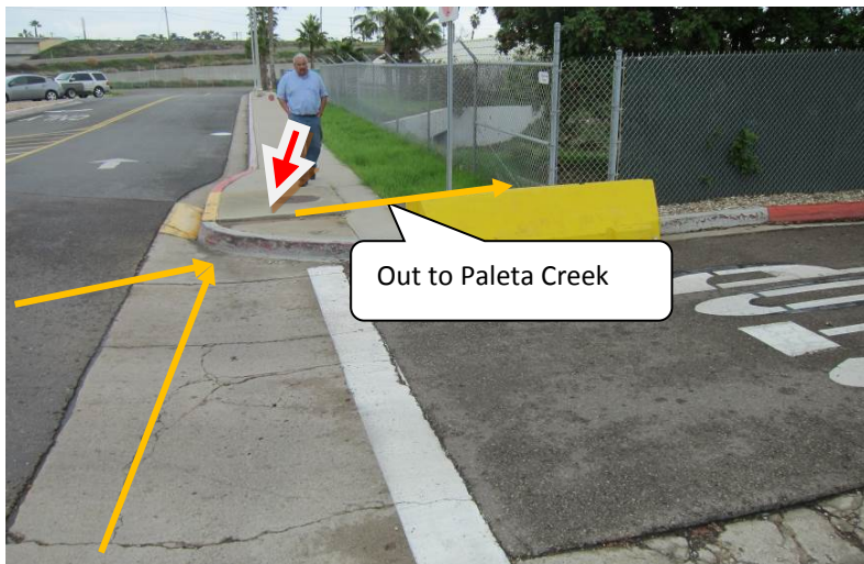
Photo of Outfall Sampling Location #4 looking east. Two storm drain pipes and curb runoff converge at the catch basin indicated by the red arrow. Orange arrows indicate direction of flow.
