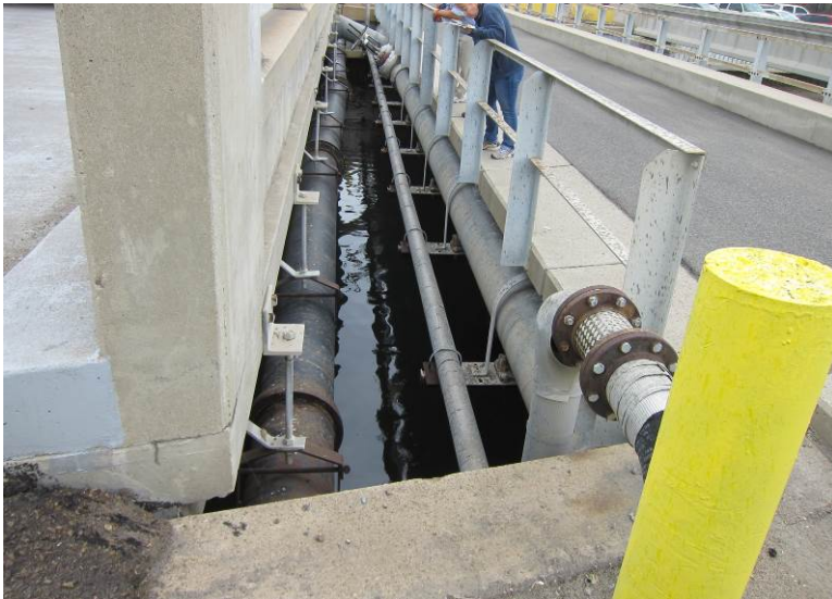
Photo looking north from potential sample equipment staging location.
