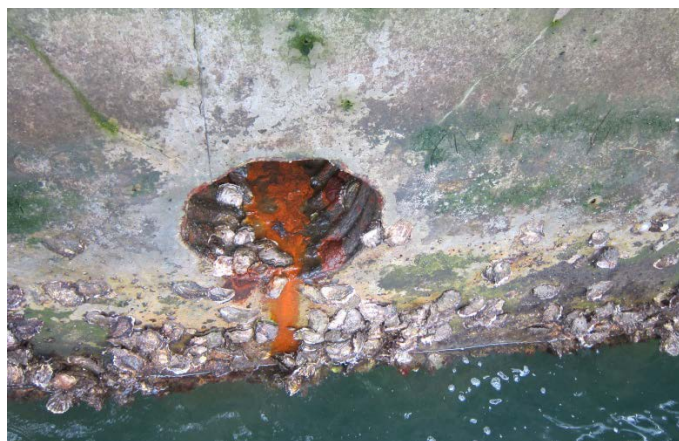
Outfall from Stormdrain #33 into Paleta Creek. Ground surface to bottom of CMP – 8'3". Rust evident in pipe. High tide water mark on concrete wall approximately 3' above top of discharge pipe. Access to discharge by boat only.
