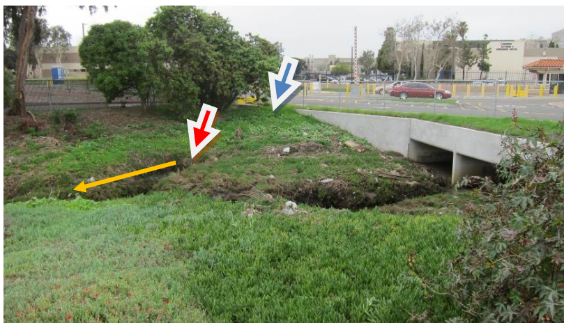
Outfall from Sampling Location #4 into Paleta Creek indicated by red arrow. Orange arrow indicates direction of flow. Blue arrow indicates approximate location of catch basin.
