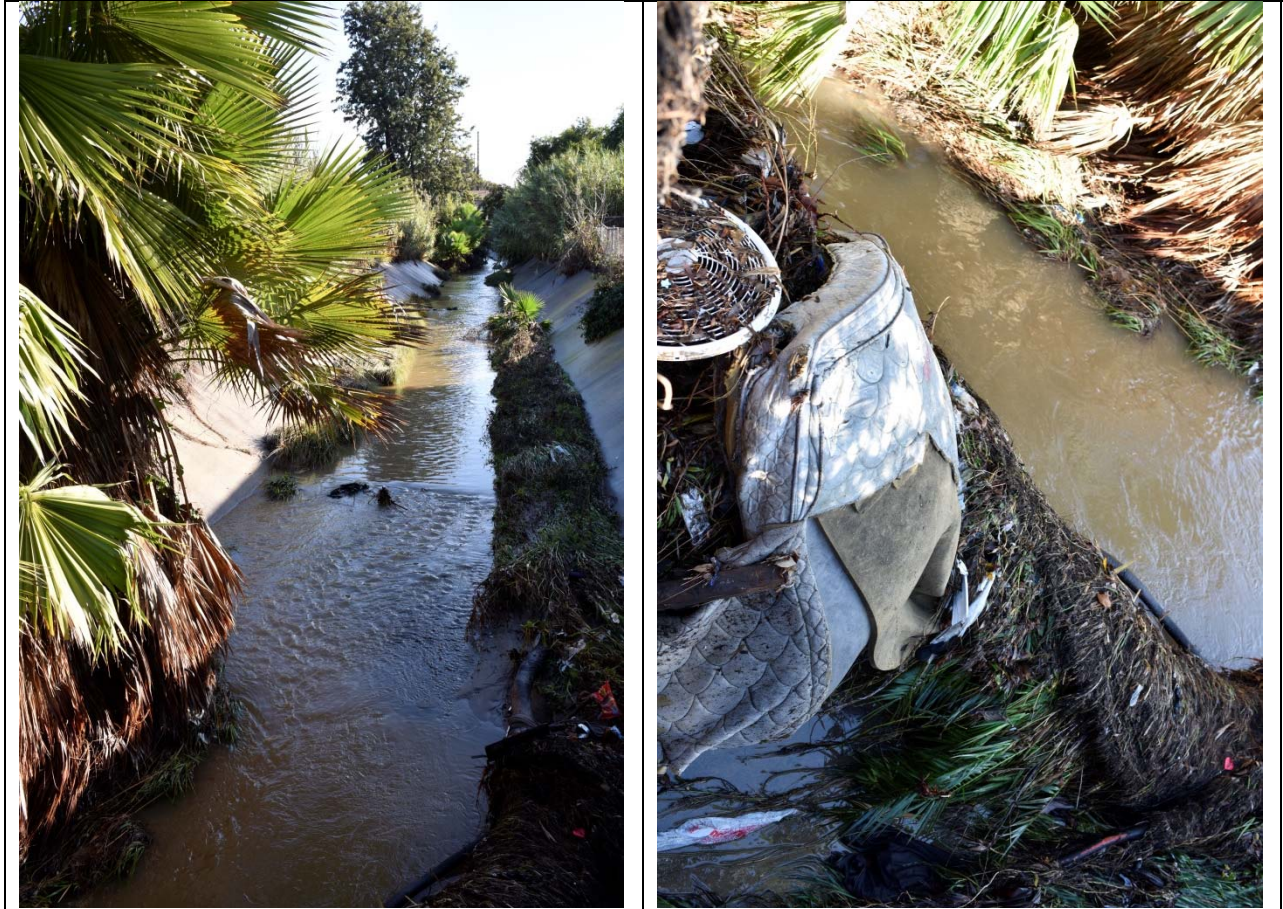
Also channelized with lots of stable sediment and vegetation. Upstream side of culvert crossing caught large debris (mattress, fan, etc.)
