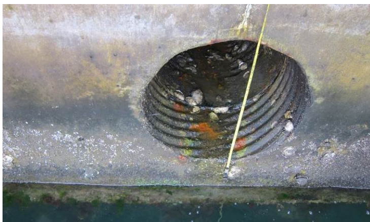
Outfall from Stormdrain #23 into Paleta Creek. Ground surface to bottom of CMP – approximately 7'. Rust evident in pipe. High tide water mark on concrete wall approximately 18" above top of discharge pipe. Access to discharge by boat only.
