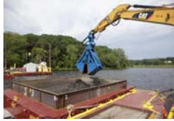
Dredging on the Hudson River
