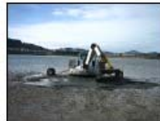
Aquamog Mixing Activated Carbon Slurry
