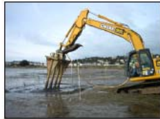
Rake Injector Mixing Activated Carbon Slurry
