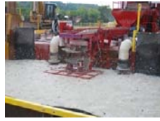
Capping on the Fox River
