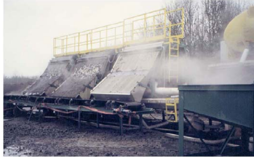
Figure 2. Wedge wire screens in parallel discharging to conveyor
