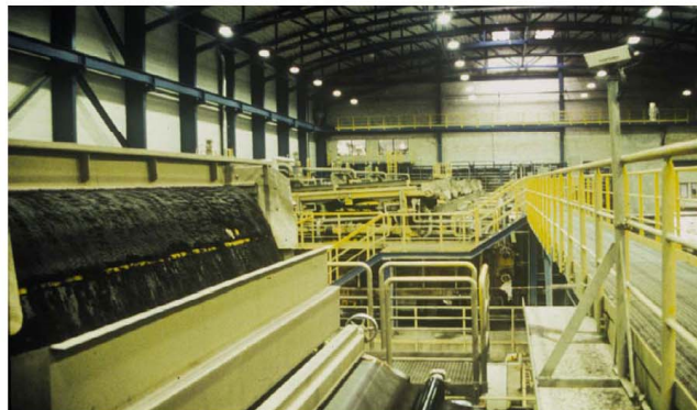
Figure 4. Parallel press installation and cake discharge
