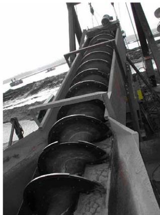
Figure 1. Sand screw preceding conveyor
