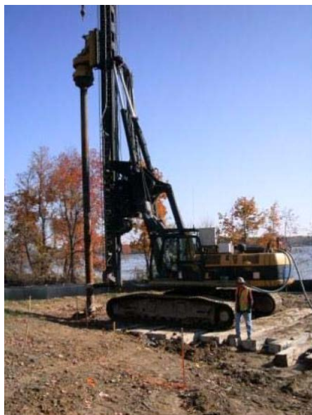
Figure 8. Soil Mixing Equipment at Site 17 (CH2M HILL 2013).
