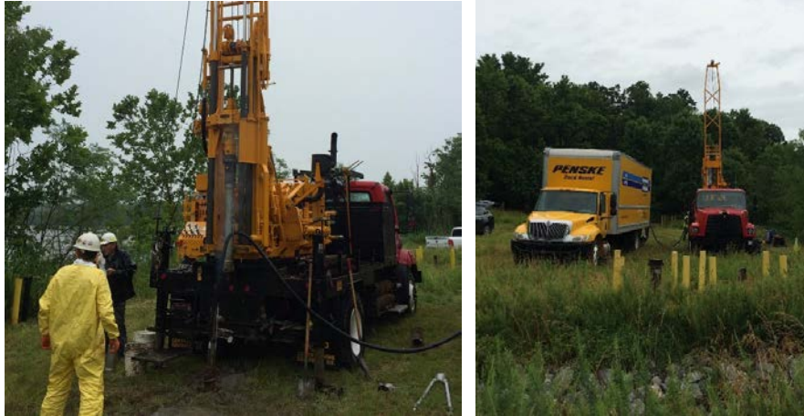
Figure 15. Photos of Hollow Stem Auger Rig and Support Vehicle Used for Cryogenic Coring.
