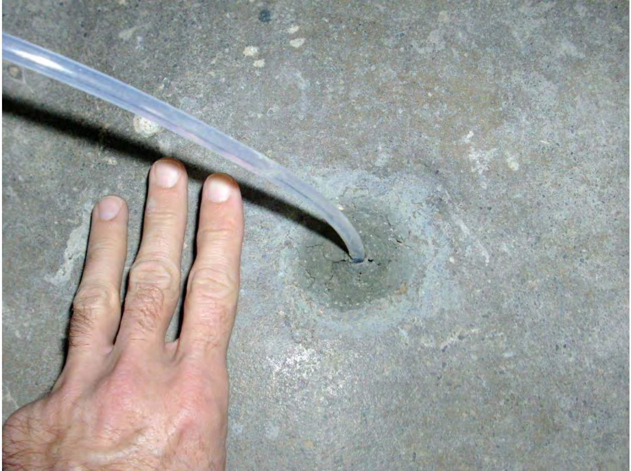
Temp Port 3 close up
