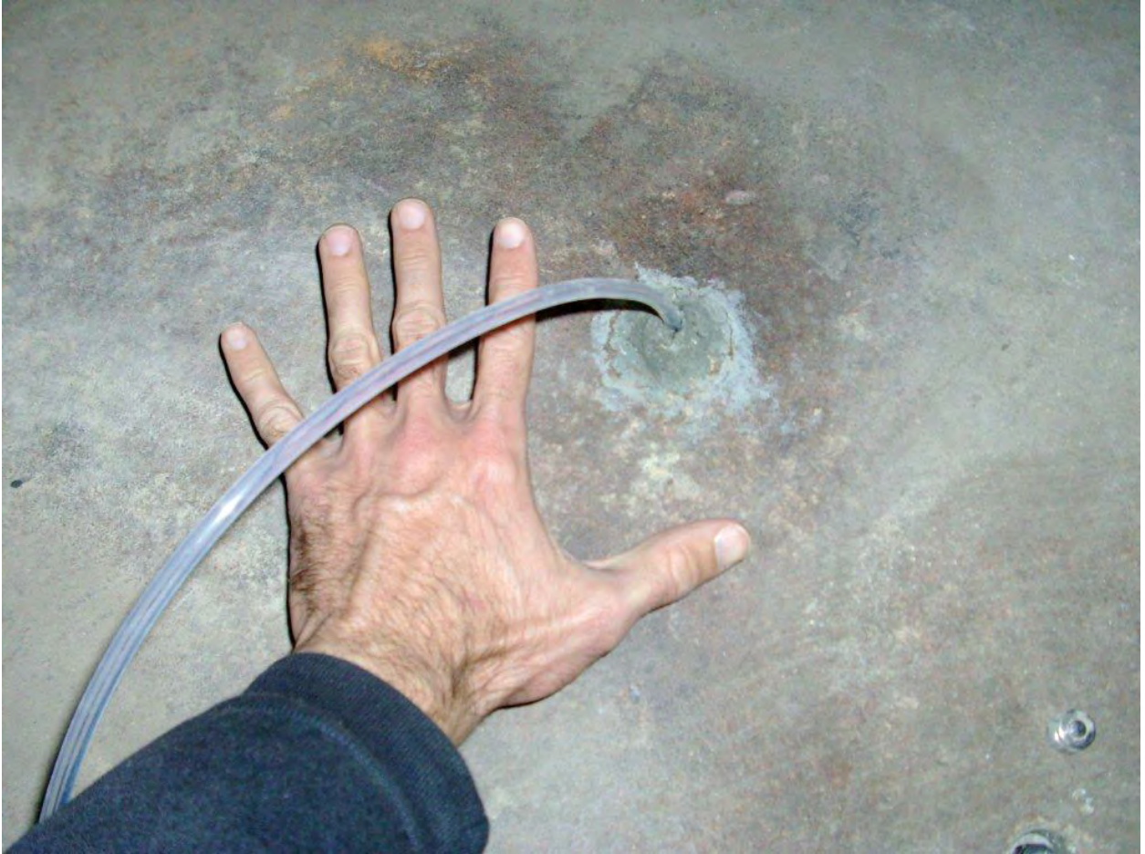
Temp Port 5 close up
