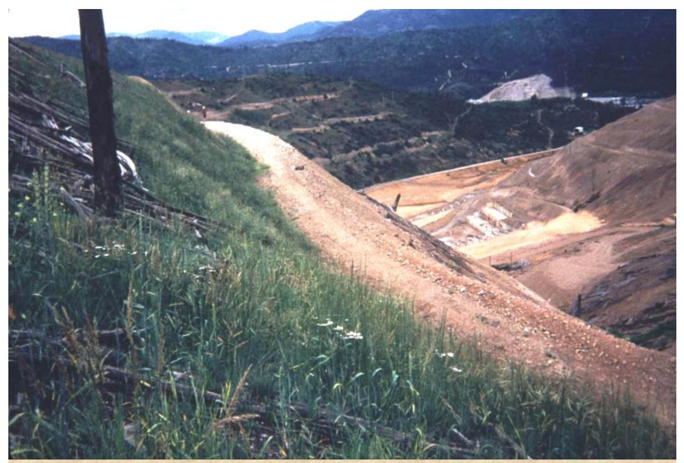
Revegetation of Bunker Hill Hillsides using mixture of biosolids, woodash and logyard debris, after 2 years.
