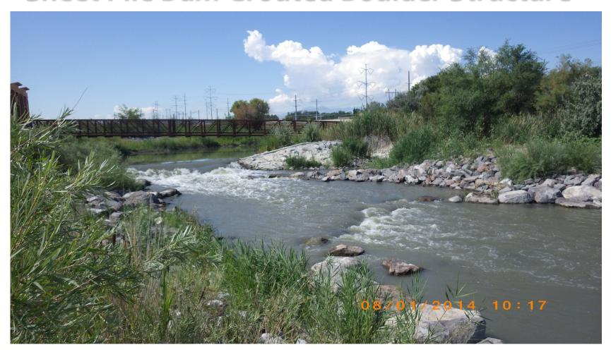
2014-Grouted boulder structure repaired with two added cross-veins to aid in navigability
