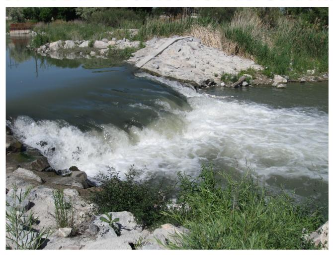
2010 and 2011- High Flows cause damage to the grouted boulder structure
