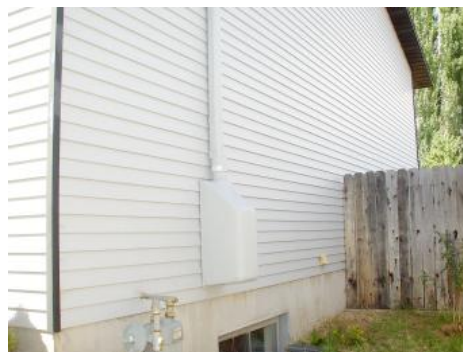
A sub-slab depressurization system is an effective, proven way to keep chemical vapors from entering the indoor air of homes.
