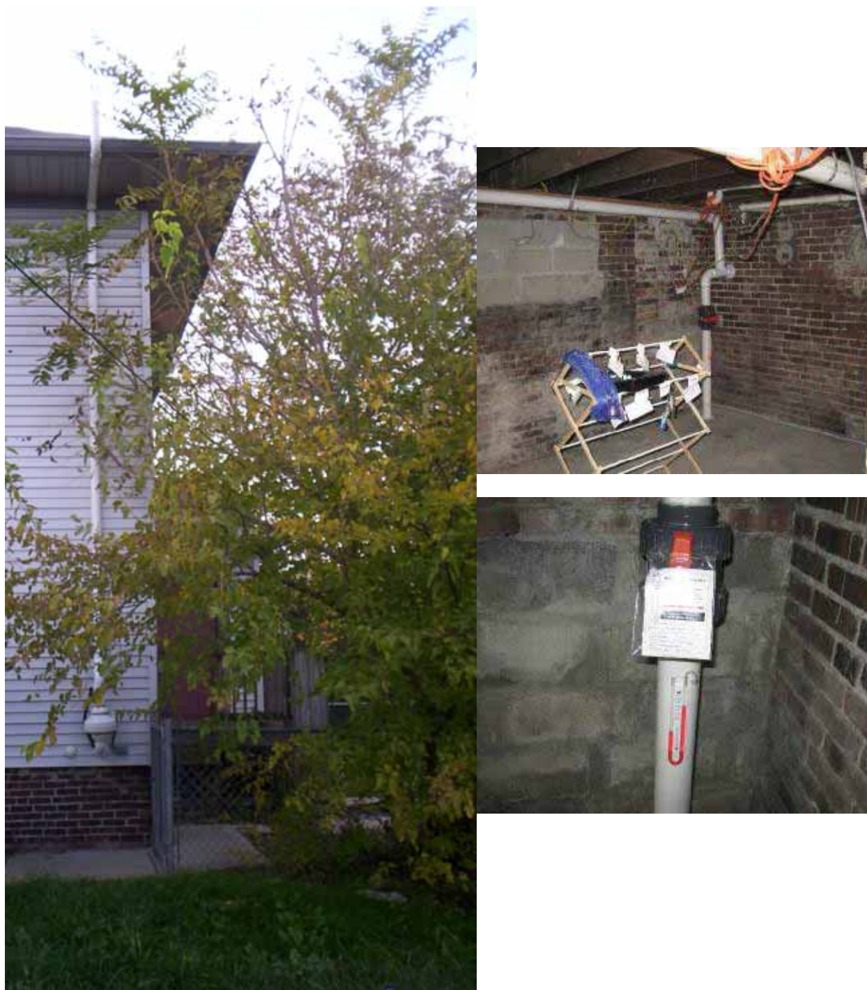
Figure 3-12. Photos of mitigation system: (left) SSD blower and stack on northeast corner of duplex; (right) SSD extraction point, showing valve and U-tube manometer.
