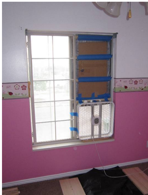
Figure 7. Fan Installed for Building Pressure Control at the ASU House.
