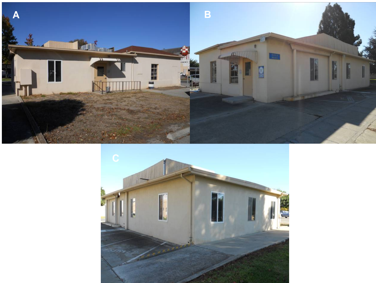
Figure 4. Photographs of Moffett Field Building 107. Panel A Shows the West Side of Building, Panel B the Southeast Corner, and Panel C the Northeast Corner.
