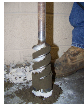
Figure 3. Suction point installation.
