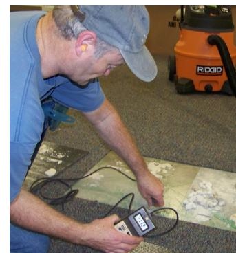
Figure 5. Measuring sub-slab vacuum.
