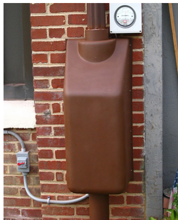
Figure 7. Low-pressure vacuum gauge and sensor.
