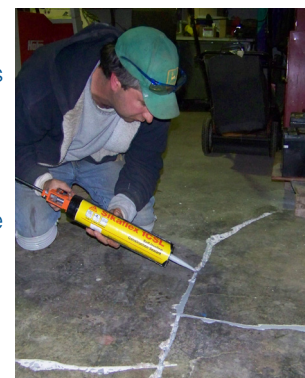
Figure 1. Sealing floor cracks.
