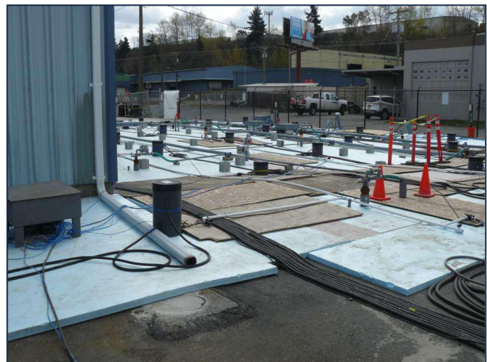
Figure 4. Well 12A ISTR electrodes at 15- to 17- foot spacing
