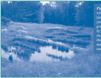
Figure 4. Circulation within the wetlands (as depicted after one year of vegetative growth) is enhanced by inner berms to increase the length of the flow path and maximize residence time of MIW.
