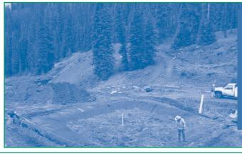
Figure 2. The biochemical reactor occupies a 35- by 35-foot area approximately 200 feet from the mine adit and 25 feet upgradient of the aerobic polishing cell.
