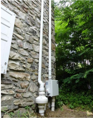
Figure 2. Typical residential exterior exhaust stack for a sub-slab depressurization system near the Crossley Farm site.
