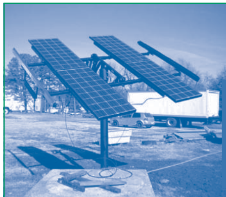
Figure 2. The passive solar tracking system at Busy Bee Laundry relies on transfer of a fluid (freon) from the east side to the west side of the PV mounting rack, as the sun continues to heat a reservoir throughout the day.
