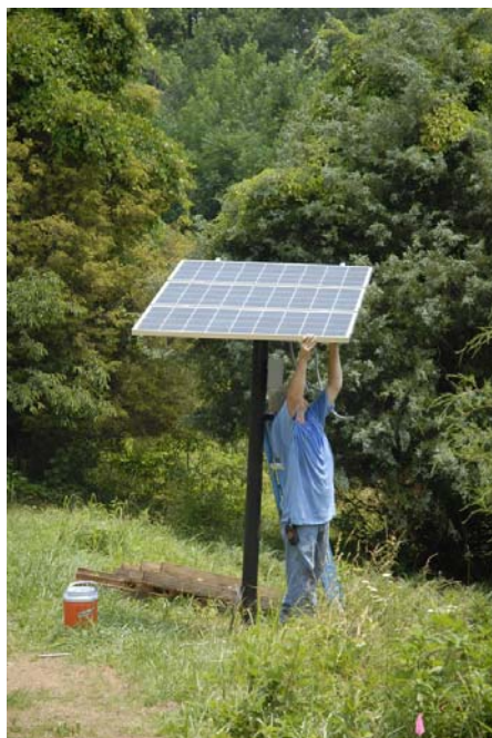
Figure 3: PV Array at Crozet Site
