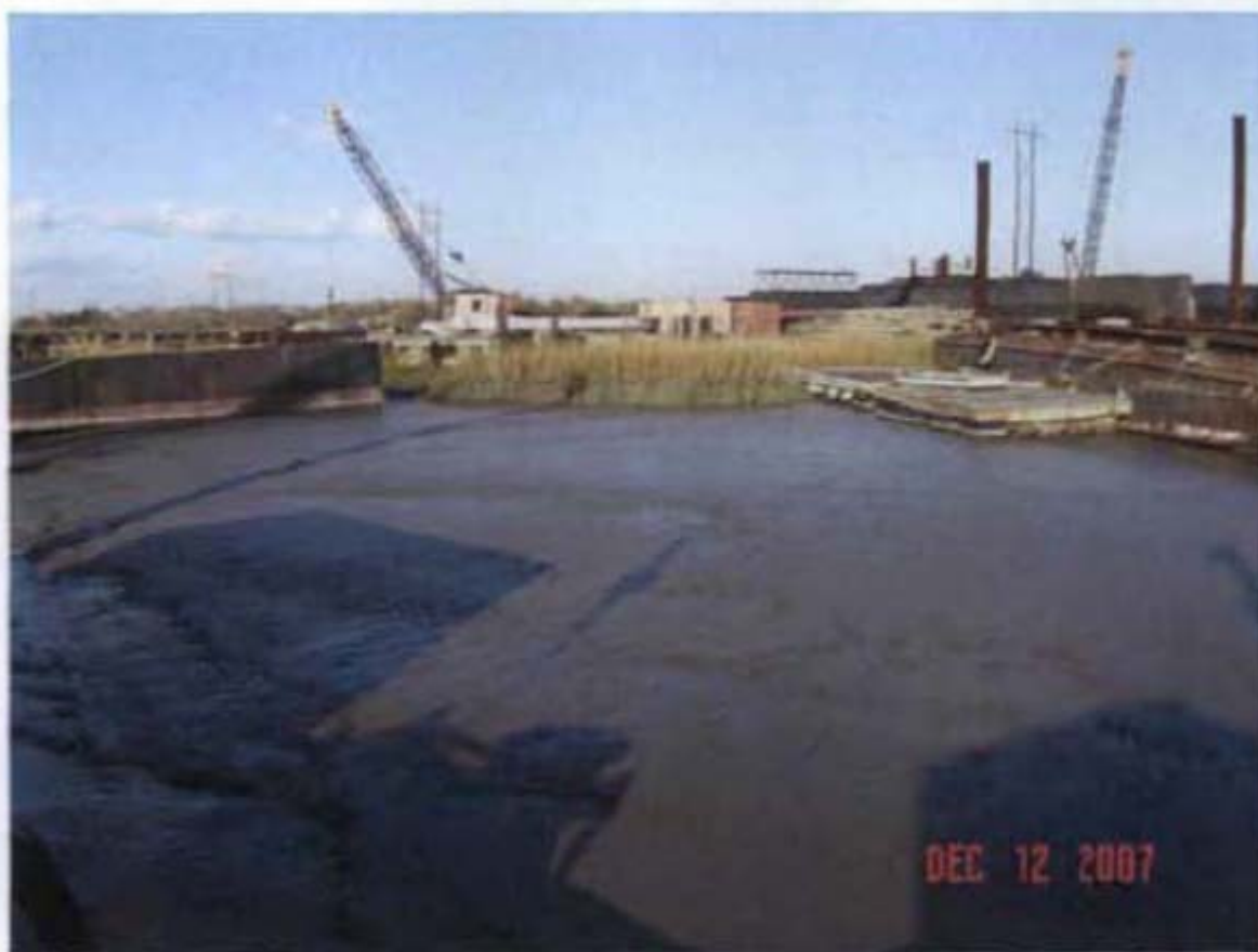
Solidified/Stabilized Section of Ashley River Cap
