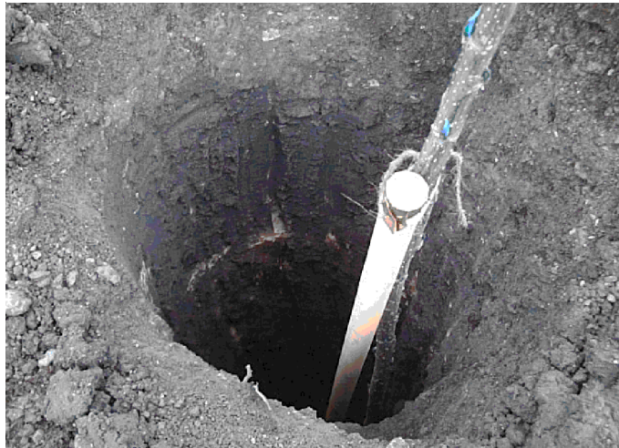
Figure 2. 10 ft hole augered through soil, rock, and concrete at Ashland site, 2000 (Photo courtesy of Ecolotree)
