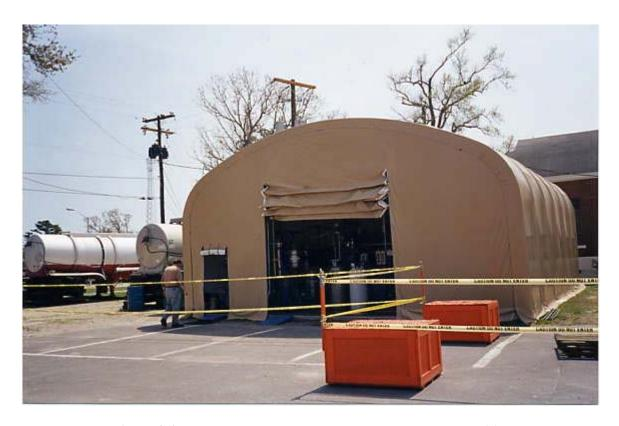
Figure 3-3. Temporary Tented Wastewater Treatment Facility
