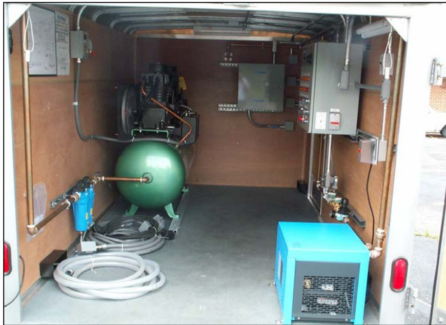
Figure 5.3. Inside of Trailer #1 – Controls and Air Supply System.
