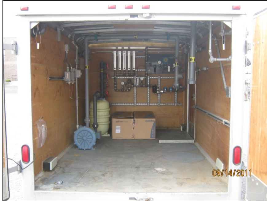
Figure 5.4. Inside of Trailer # 2 – Propane Feed, and Distribution and SVE Equipment.
