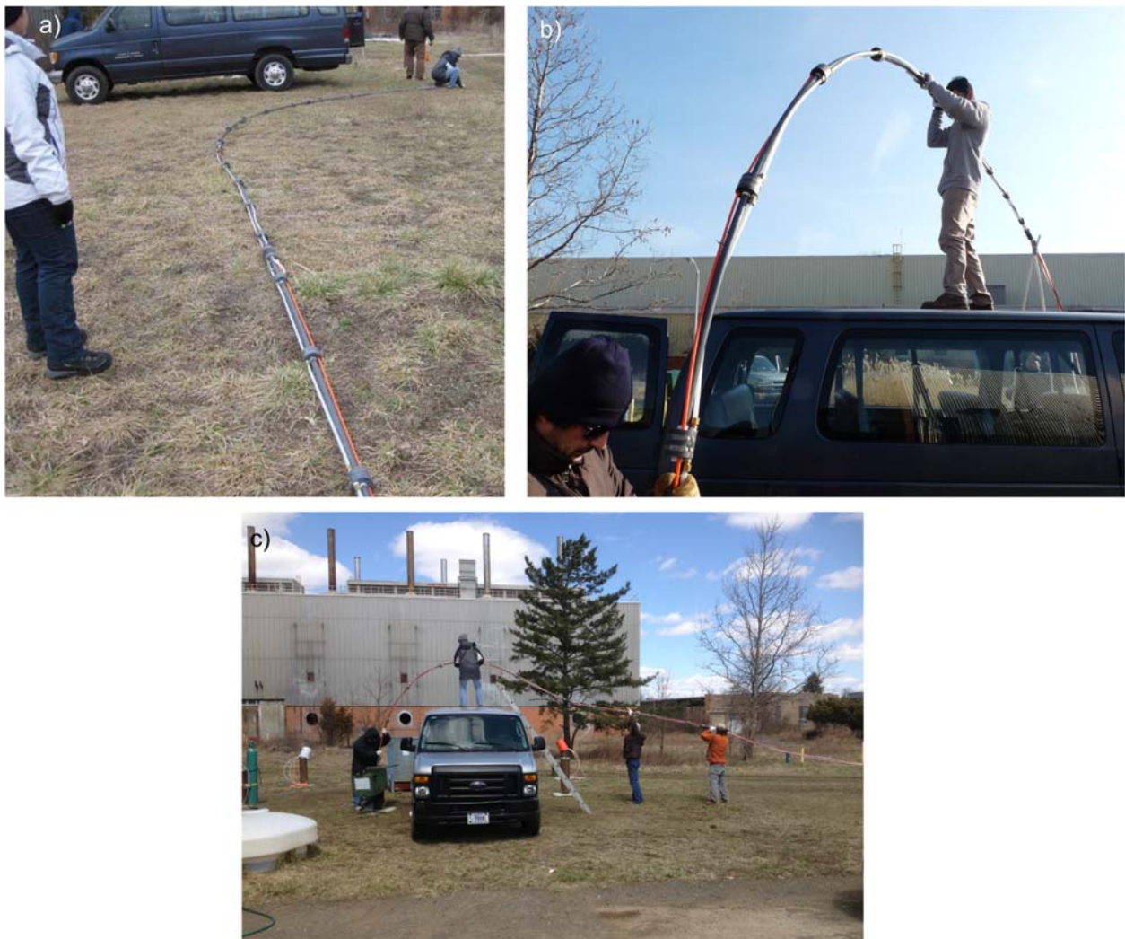
Figure 5.4.10: a) Assembly and ground testing of electrode array at NAWC b) Installation of electrode array into borehole c) Five person crew installation of electrode array.
