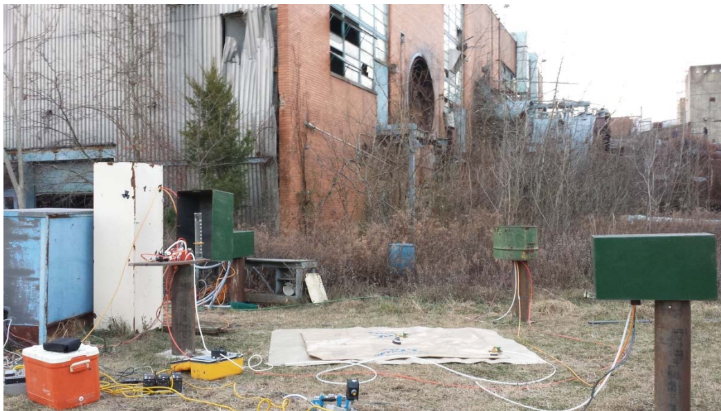
Figure 5.5.3 1: Extraction of native groundwater from 83BR into a 200-gallon bladder on the surface. The center well with the extraction tubing and peristaltic pump is 83BR.
