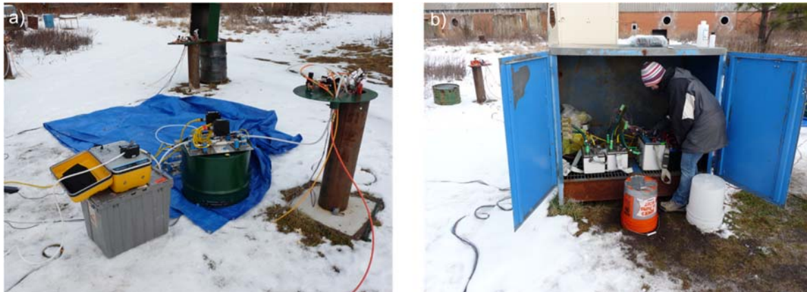
Figure 5.5.3 2: a) Extraction pumping from 85BR after injection of a conductive fluid and native groundwater in 83BR b) ERT data collection
