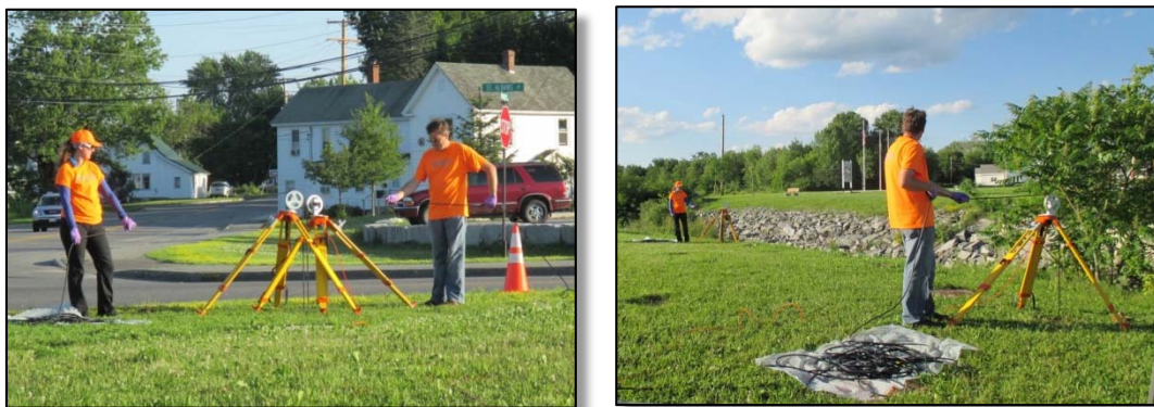
Figure C.3: Borehole GPR collection in EWM BM38 single mode (left) and level run between BM32 and BM35 (right)
