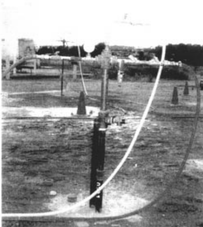
Figure 3. Photo of Geo-Cleanse® injection well.
