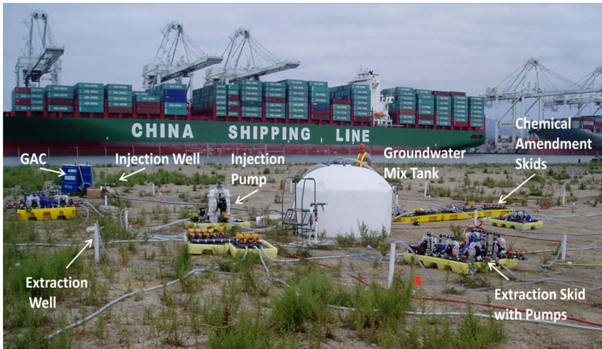
Figure 5-7. Injection and Extraction Equipment
