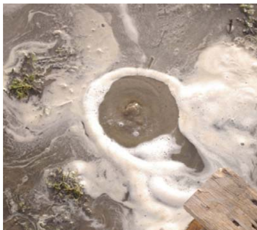
Figure 5-18. Daylighting During ISCO Injections
