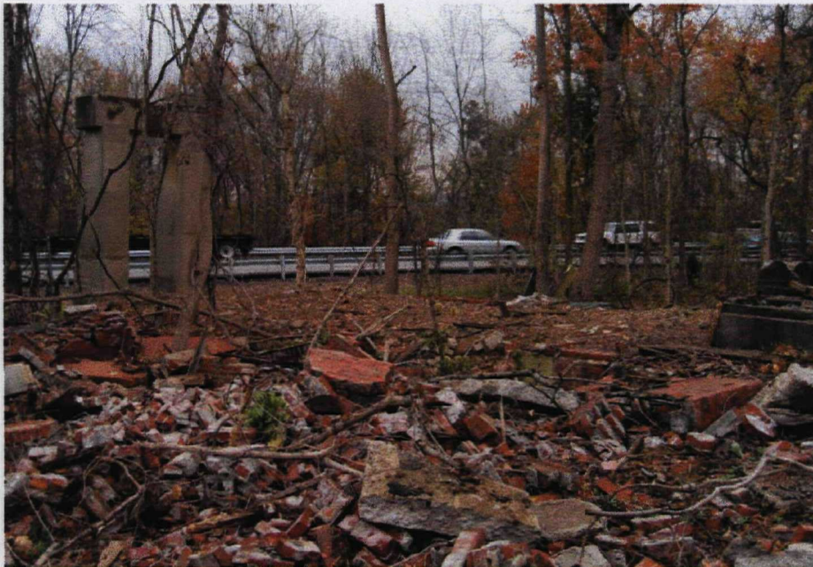
Debris, including bricks and concrete, from the brick kiln and warehouse demolition along Dixie Highway at the Distler Brickyard site.
