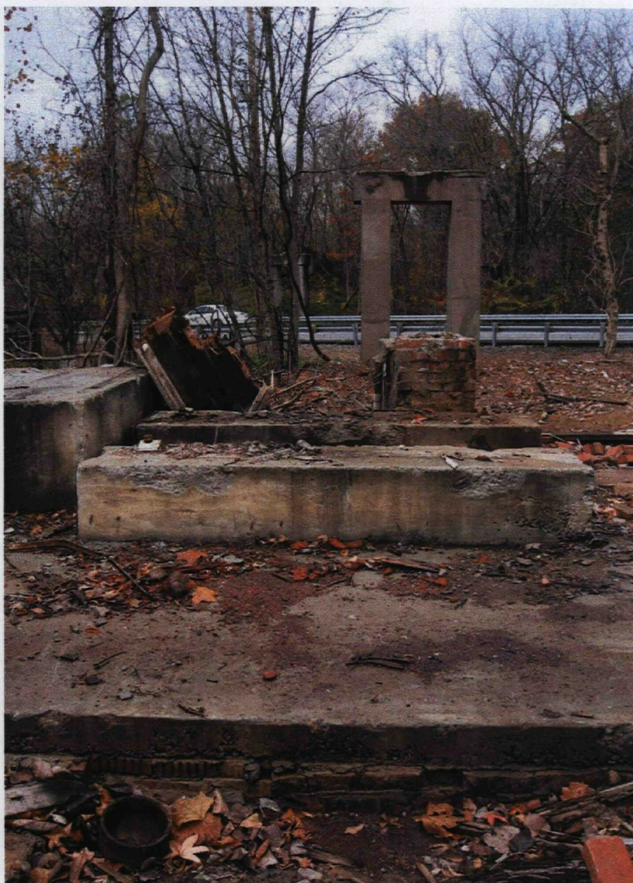
Remnants of warehouse foundation and bridge over Dixie Highway.
