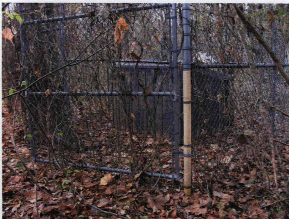
Fenced pump and treat system.
