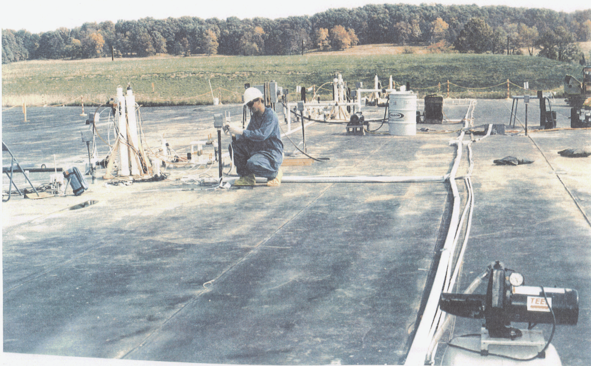
Figure 2.5. Photograph of the established demonstration test area at the X-231A site.
