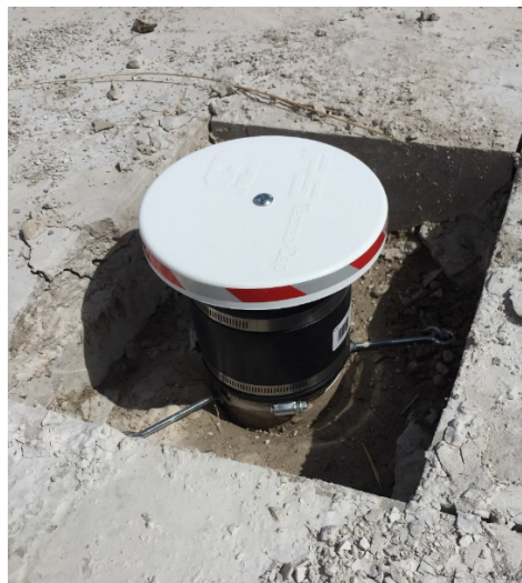
Figure 5.2. Carbon Trap (E-Flux) Installed within a Paved Location at TEAD-S.
