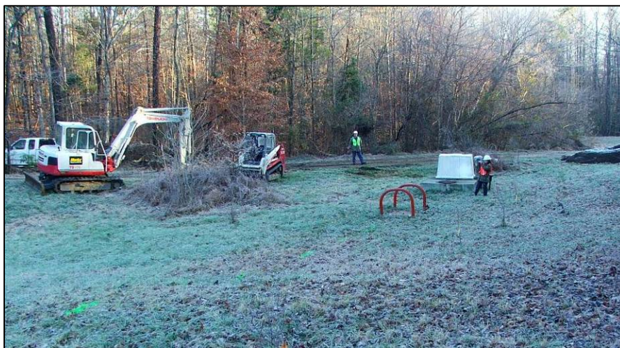
Figure 2. 12/05/05. Site appearance before installation of EBuffer®. Temperature was 20 degrees Fahrenheit. Approximately 1.25 inches of rain had fallen the previous day.
