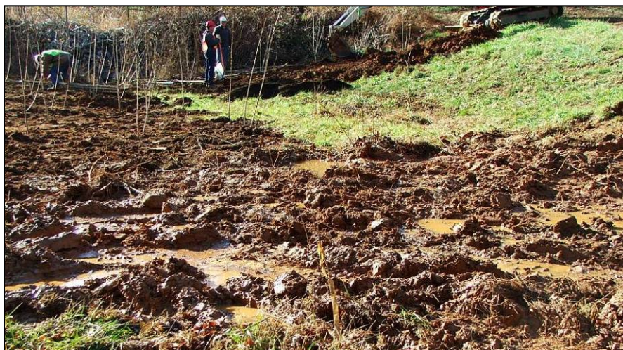
Figure 3. 12/05/05. Water on the site was runoff draining from the landfill following the previous day's rain. It did not stop the installation.
