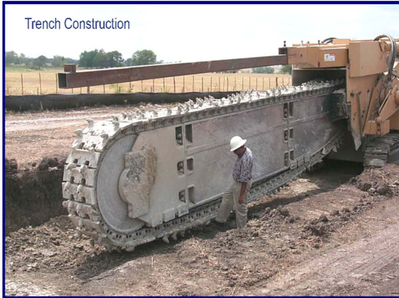
Figure 4-3. Rock Trencher Used for Biowall Installation at McGregor, TX
