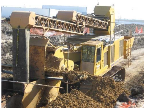
Figure 2-2. Rock Trencher Used to Install PRBs at NWIRP Dallas, TX
