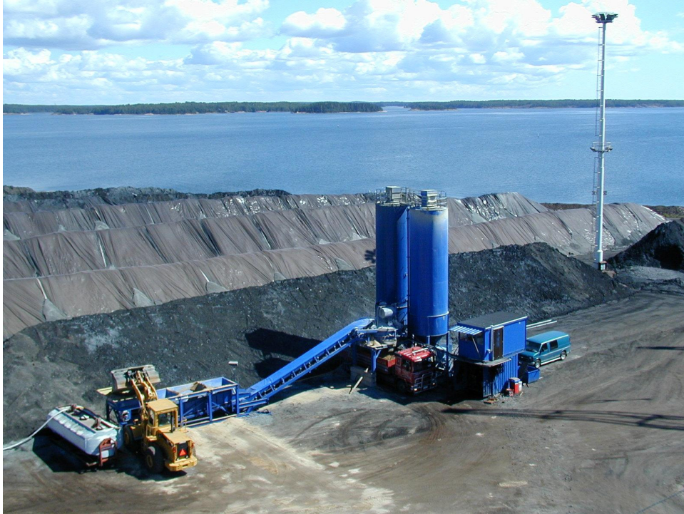
Figure 20: Ekomen system to mix and stabilize/solidify inorganic contaminated soils. The equipment is movable to the treatment site. (Ekokem / Österbacka)
