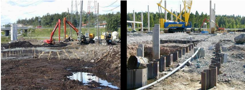
Figure 14. Photos of the on-going foundation works at the IKEA site (Koivisto et al. 2004)
