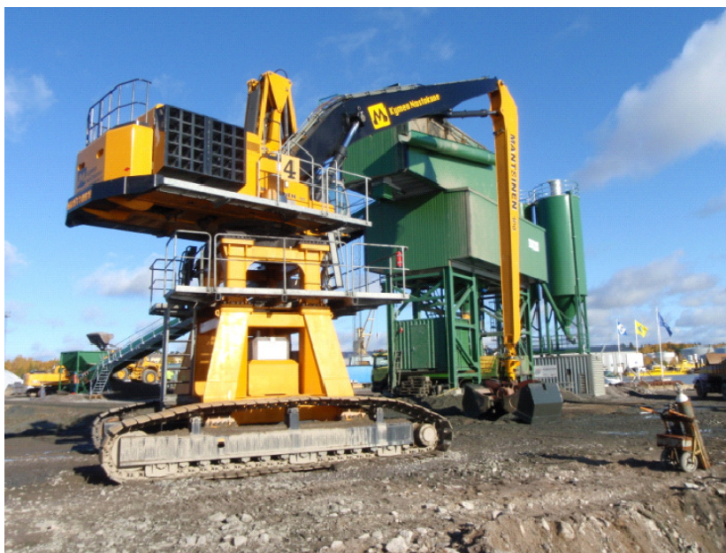
Figure 8. The picture shows process stabilization unit (approx. capacity 200 m 3 /hr). The binder is fed into the mixing chamber by the conveyor belt to the left and from two silos. The grab-dredger feed soil and sediments into the chamber on the top.
