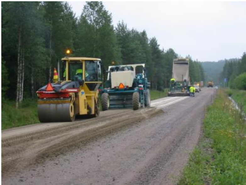
Figure 26: On-going stabilization in Rautavaara in 2004, on the left lane of the road. In front goes the lorry and asphalt spreader for the binder. After this come the stabilization cutter and the first compacting roller (Ramboll Finland Oy).
