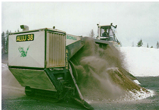
Figure 1: Mass stabilization with stack mixing of excavated soils or by-product materials. Method is applicable for all types of soil.
