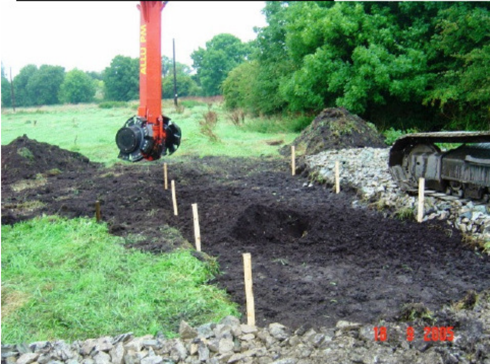
Figure 15. Test field for deep stabilization of Irish peat in September 2005. (Niutanen 2006b)
