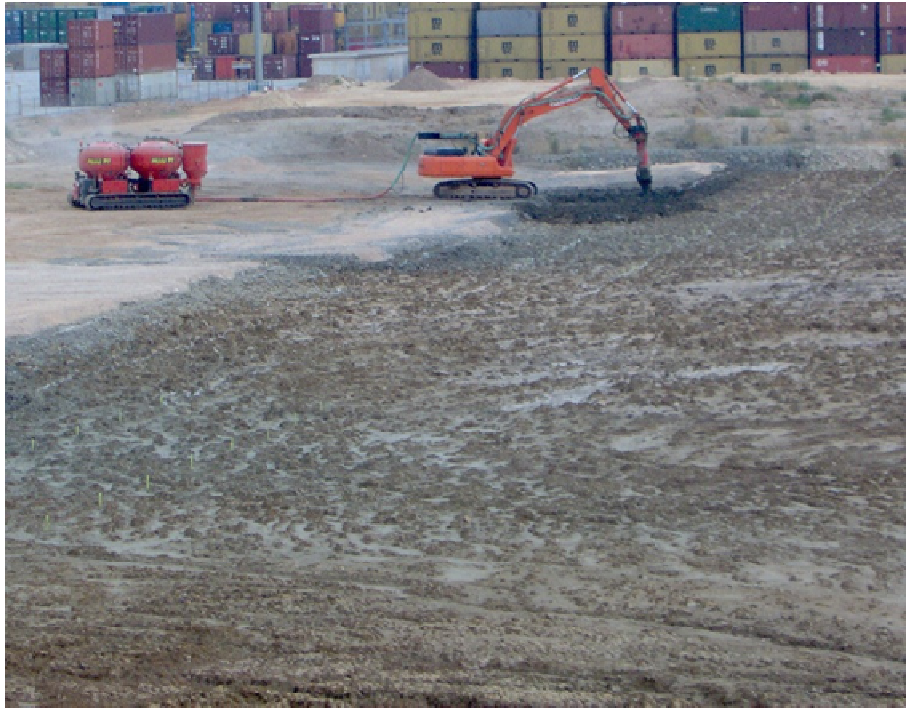
Figure 18: On-going works of test stabilization. Spain 2005 (Niutanen 2006a)
