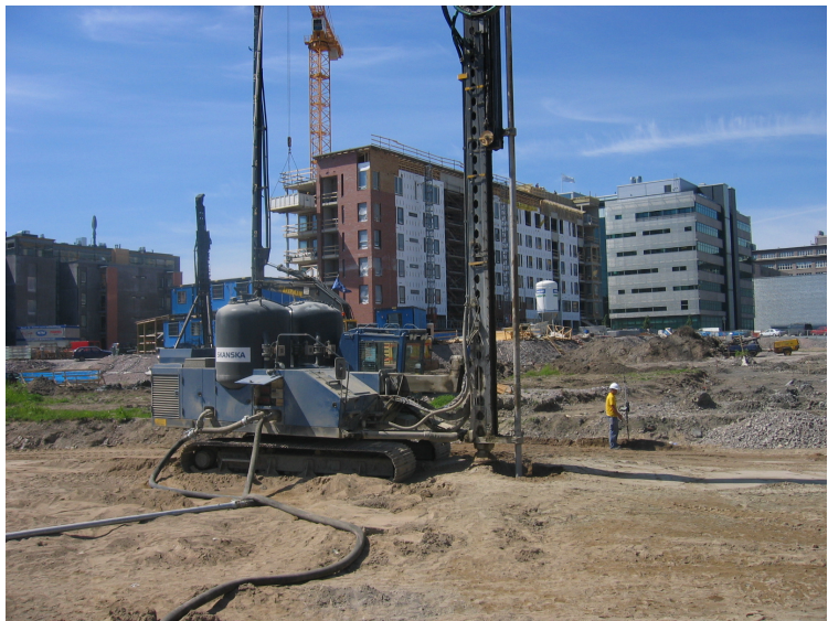
Figure 11. Five sections of column stabilized zone wall of Arabianranta, Helsinki (2000-2005). The wall stiffens and strengthens making a retaining wall. (Forsman et al 2006)
